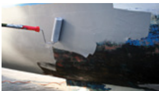
Apply Underwater Primer onto prepared surface
