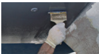
Lay off Gel/High Protect in opposite direction with brush
