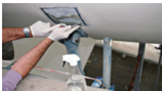
Wet scrape to remove old antifouling
