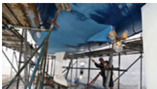
Clean abraded surface
