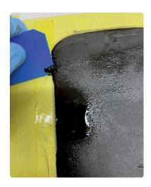
**Step 8:** Immediately peel off the masking tape and use tape to hold the cover plate in place if necessary.
