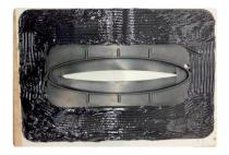
Step 6: Place the glue-coated panel under the hull and apply light pressure evenly, do not push too hard. After applying pressure, there should
