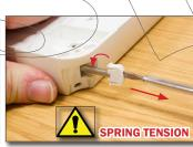
Insert screwdriver in tensioner slot and allow spring to retract from corner moulding. Spring tension will now be felt in the two directions shown.
