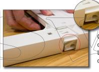
Continue to slot side rail onto corner moulding.
